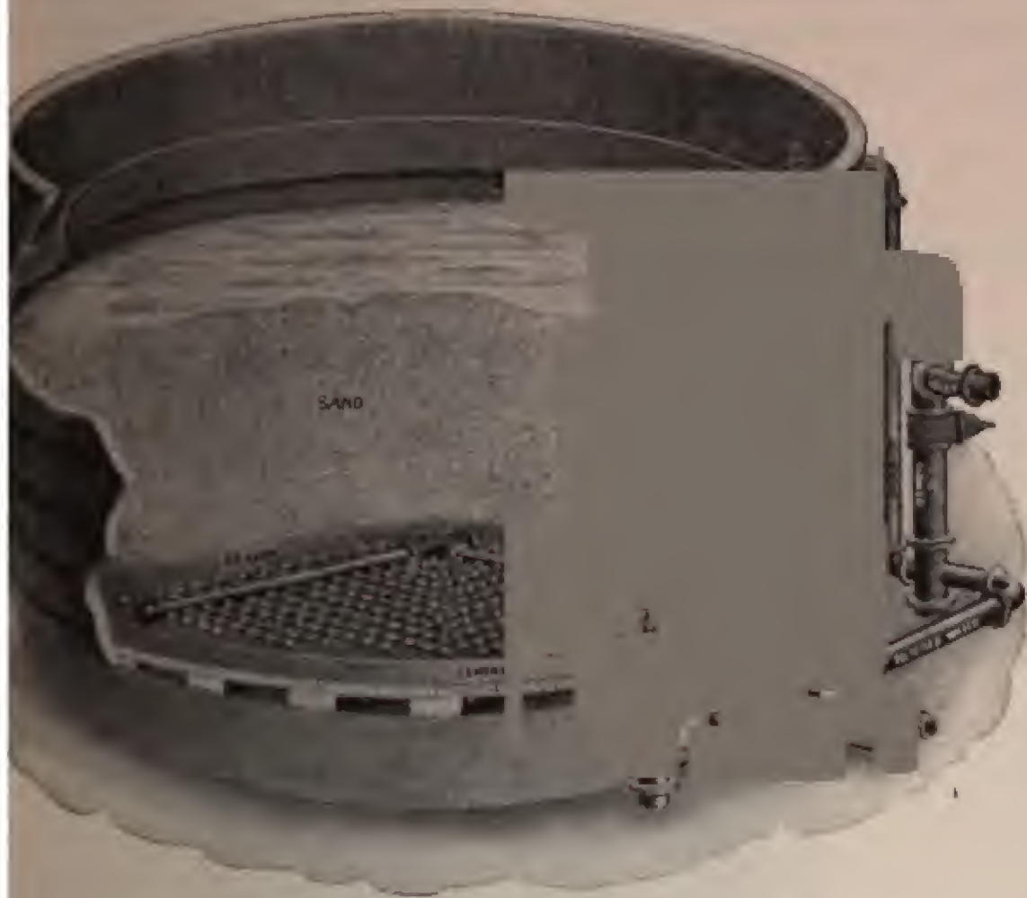
FIG. 56.—Continental "air wash" gravity filter.
